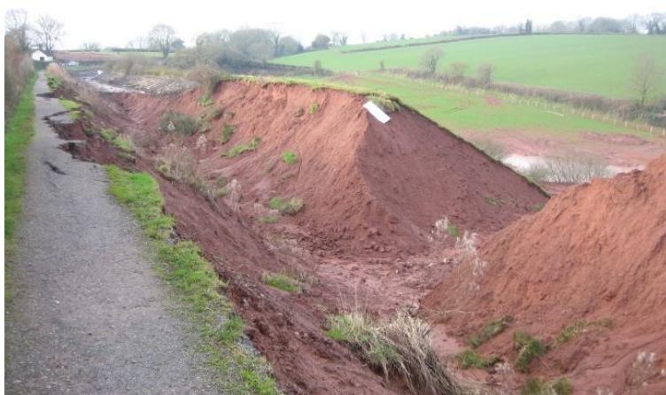
Left: Swing embankment after the 2012 breach.
